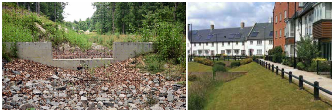
Figure 3.14: Examples of Possible Outfall Controls for the Swales
